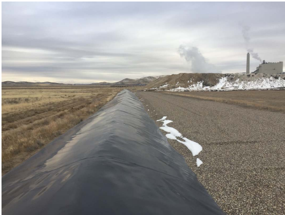
Photograph 04: East side of Cell 2 near northeast corner (looking south).
