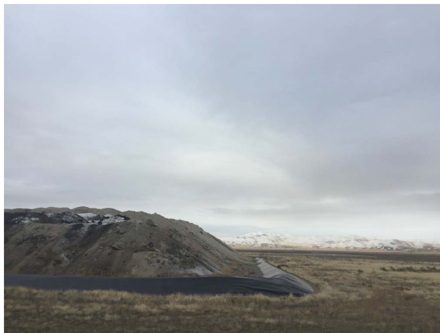
Photograph 3: East side of Cell 1 (looking north)
