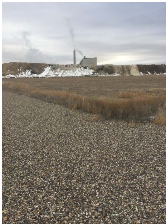
Photograph 2: Cover Material over geomembrane
